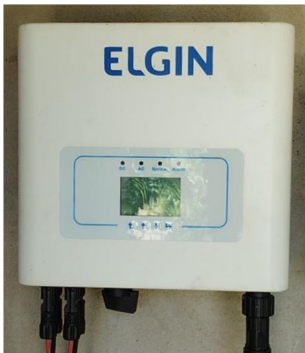
Figura 16 – Inversor Solar On-Grid
